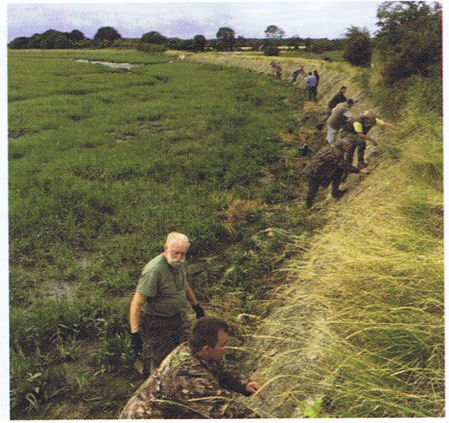
Sea wall maintenance
